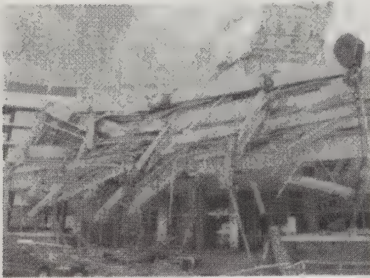
New Zealand earthquake collapse clearly indicating pancaked floors
