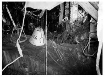
A close up view of construction "E". The cone-like objects are media monitoring sensors.
