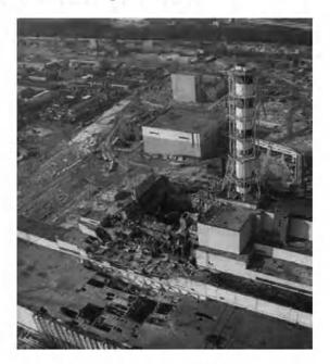
The destroyed reactor building of Unit 4, the view from the turbine room area (the southern part)
