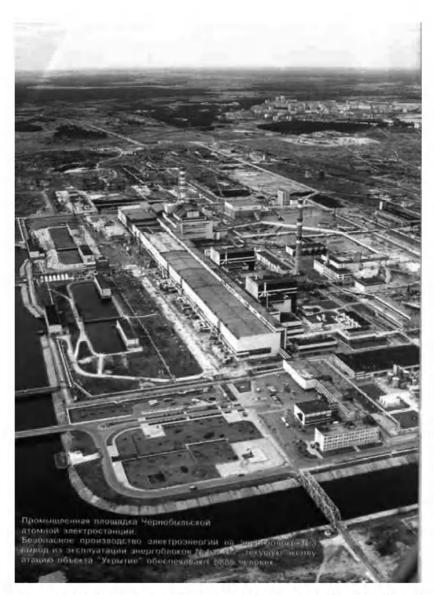
Photo of the Chernobyl NPP. The long turbine room building is visible on the forefront. Black reactor unit buildings are located behind it. The double building of reactor units ## 3 and 4 is located behind the left part of the turbine building (with the 150 m high ventilation stack between the units). The city of Pripyat is visible in the right upper corner of the photo.
