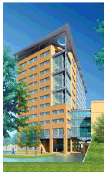
IBM's Amsterdam offices. The glass curtain walls use new coatings that reduce heat gain while providing greater visibility, to optimize interior daylight (all pictures courtesy William McDonough + Partners)
