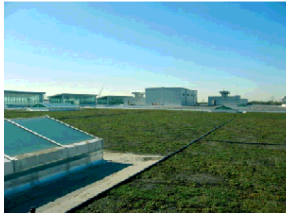
William McDonough + Partners designed Ford's new Rouge River assembly plant with the world's largest green roof.
