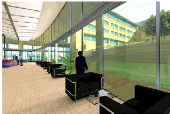
The lobby for IBM's Amsterdam offices. The glass curtain walls use new coatings that reduce heat gain while providing greater visibility, to optimize interior daylight (all pictures courtesy William McDonough + Partners)
